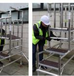
Add the additional brace below the platform. For a stepfold 2 you should now the ribbed brace. Then have 2 ribbed braces below the working
