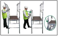
Open both end guardrails and rotate top half of side guardrail through 180 degrees (reversal of assembly procedure) ensuring that the guardrail chosen has roll pin located in the lowest slot of guardrail bracket (this enables unit to be folded in correct sequence).
